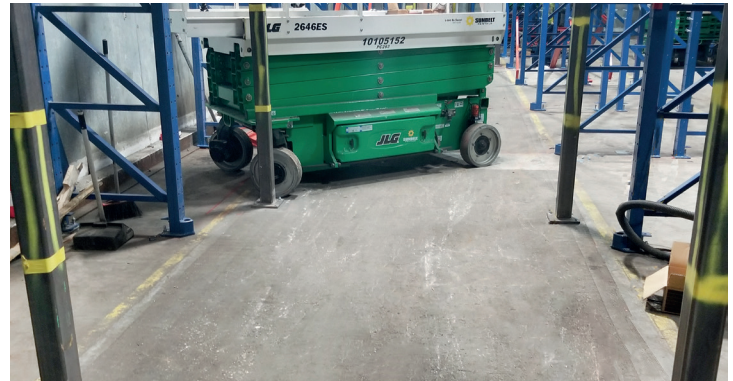
Safety First: Clearly marked temporary columns.
