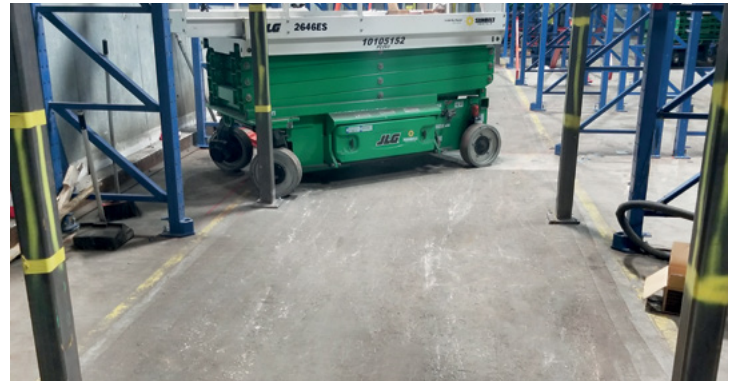
Safety First: Clearly marked temporary columns.
