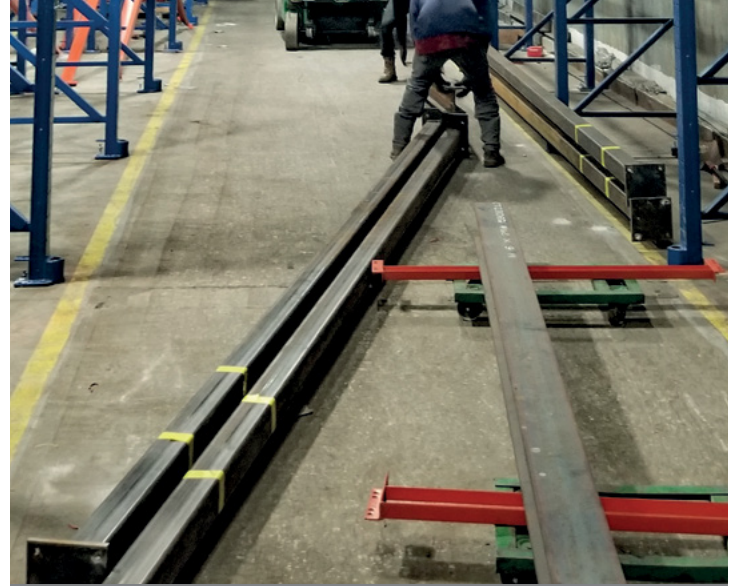
Temporary columns support ceiling while rack is dismantled & replaced row by row.
