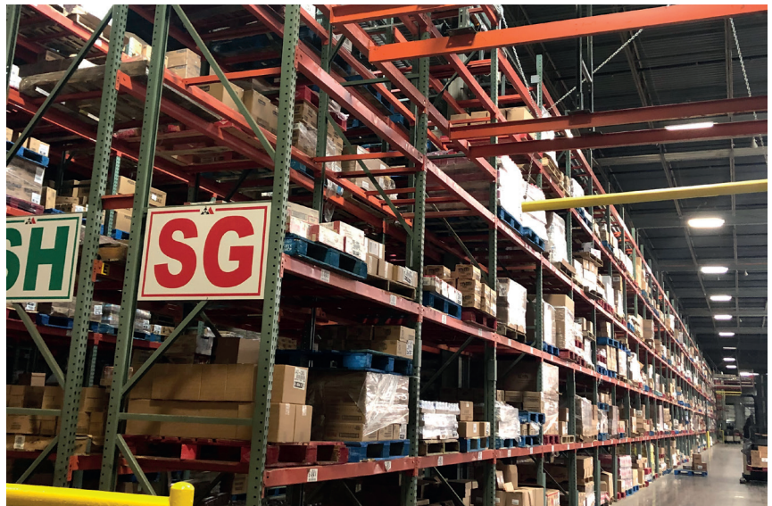
Selective rack pallet storage.
